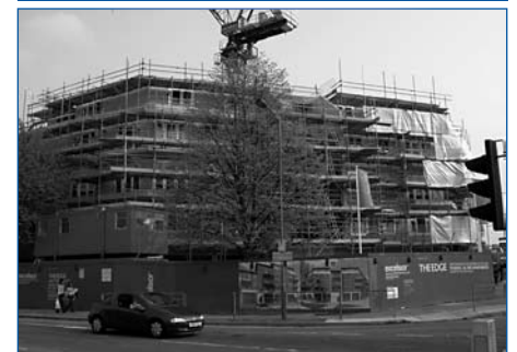
Scheme under construction
